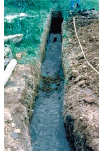
Laying SAN-EARTH M5C
