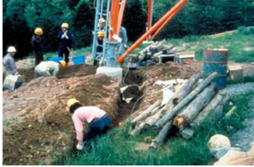
Excavation for SAN-EARTH Grounding
